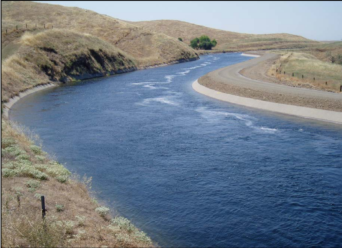
Figure 21: Friant-Kern Canal, Friant Division (Bureau of Reclamation, Jim Bailey)
