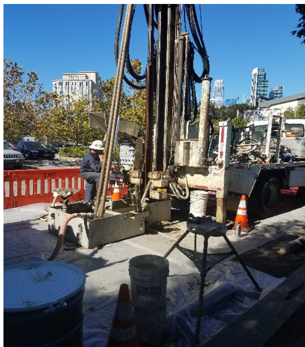
Image 3. Mud-Rotary Wash Drilling
