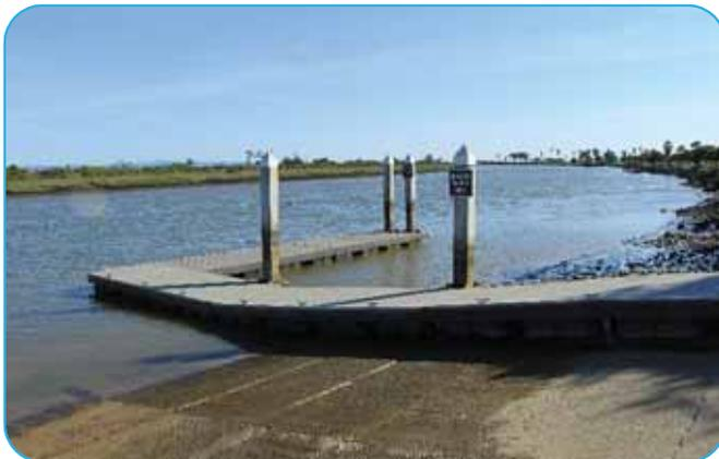
**Launch Highlights:** The right-angle design provides ample dock space and a sheltered area between the dock and the shore for non-motorized launching.
