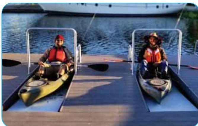
**Launch Highlights:** The two launches with grab-bars provides a stable launch and ample dock space that allows multiple users to launch or land at once.
