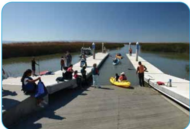
**Launch Highlights:** V-grooved concrete ramps provides an alternative launch to users that prefer not to use docks.
