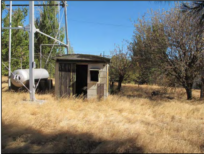
Photo 5. View of exterior of the pump house near the water tower in the central portion of the site facing north. Pump house contained one groundwater supply well, dismantled well pump, and associated plumbing, and one air compressor.
