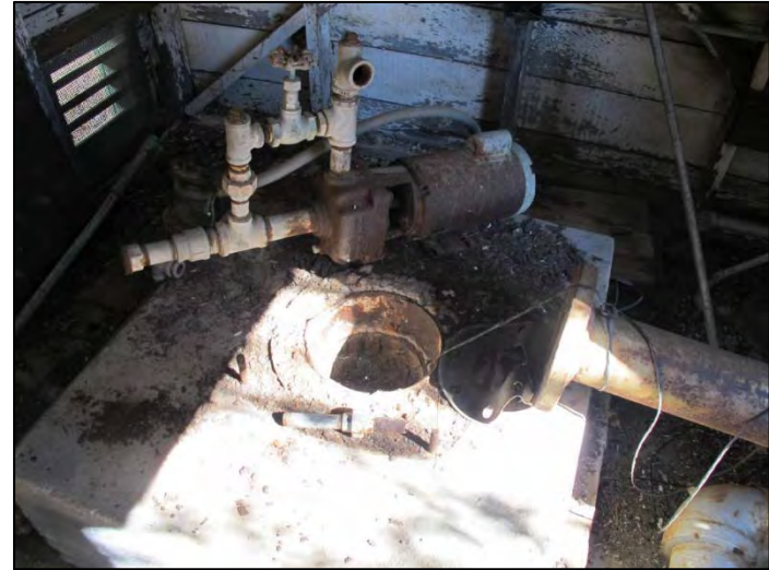
Photo 6. One 8-inch groundwater supply well with dismantled pump in the pump house. No well lid to protect groundwater was observed and groundwater level was estimated at approximately 8 feet below ground surface.
