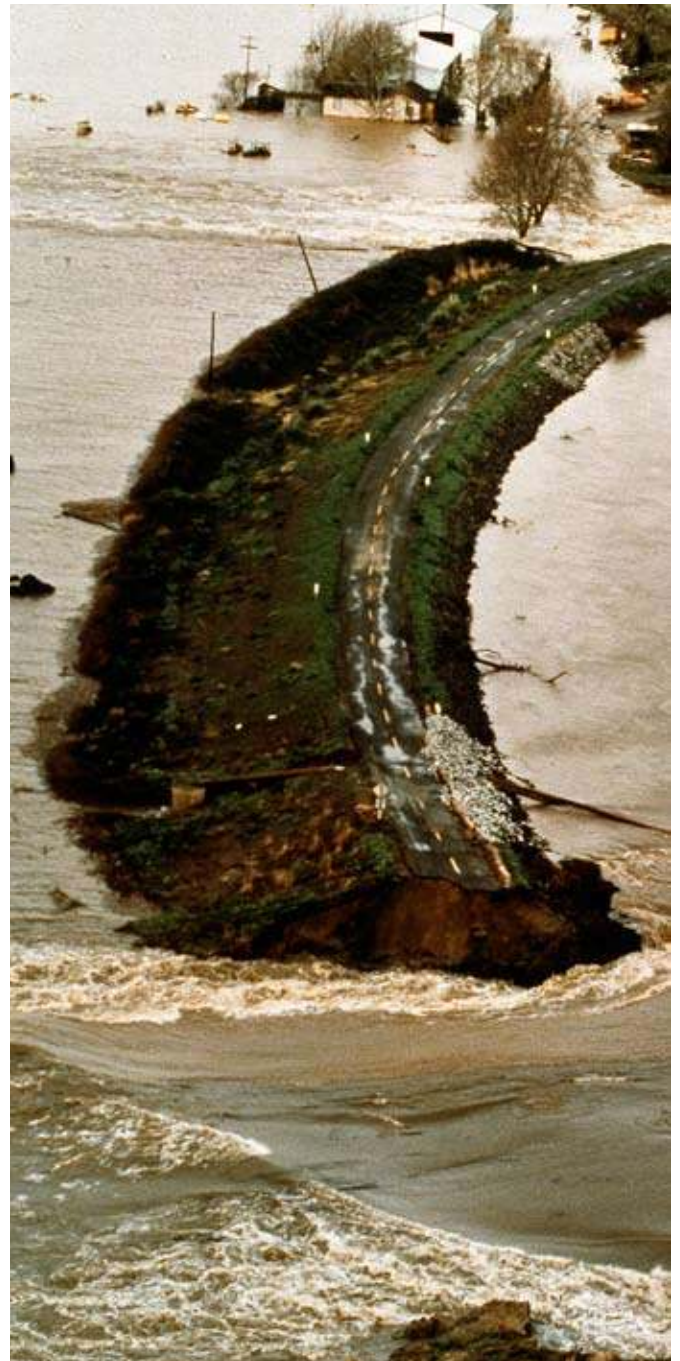
Levee breaches at Tyler Island [1986]. Source: DWR
