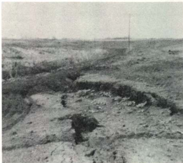
Levee damage on Bacon Island (Site 2). A 250-foot land-side rotational slip-out dropped several feet during the January 24, 1980 Livermore earthquake.
