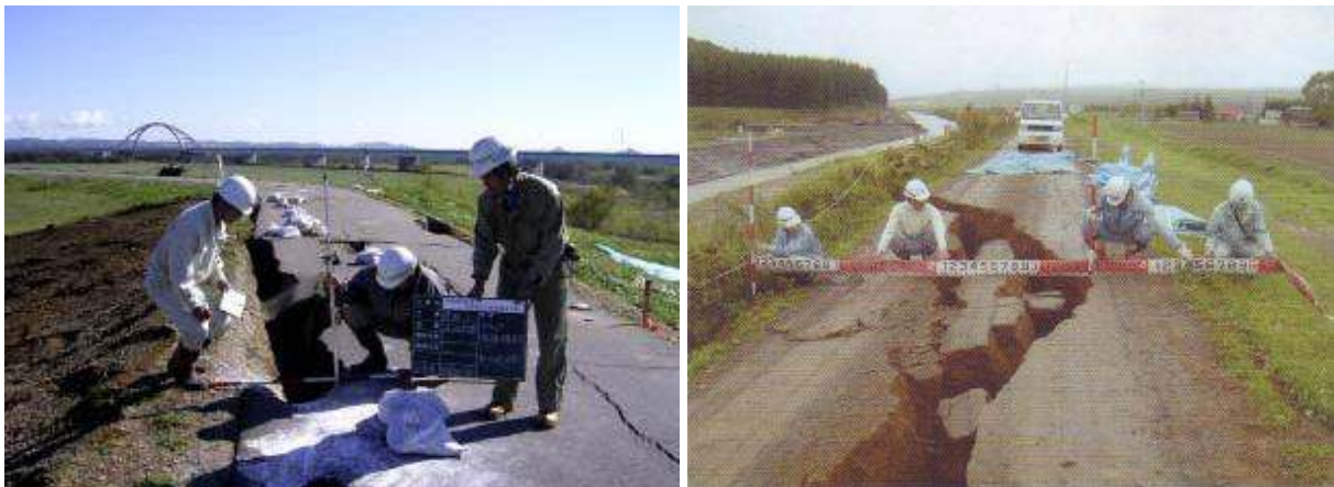
Figure 4.21 Cracking of the roadway on the levee crest accompanied by slip on the slope at Section 10.
