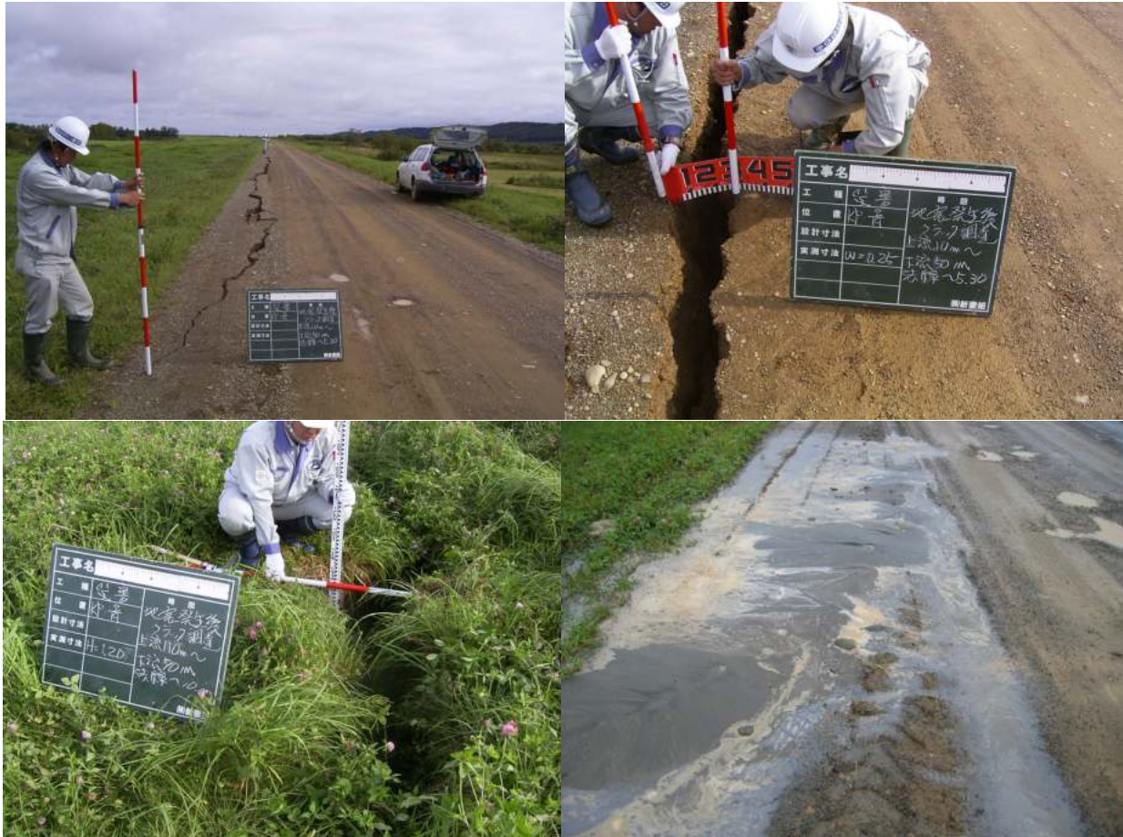
Figure 4.16 Cracking on the crest (top) and land-side slope (bottom left) at Section 8. Sand boils on crest access road downstream (bottom right).
