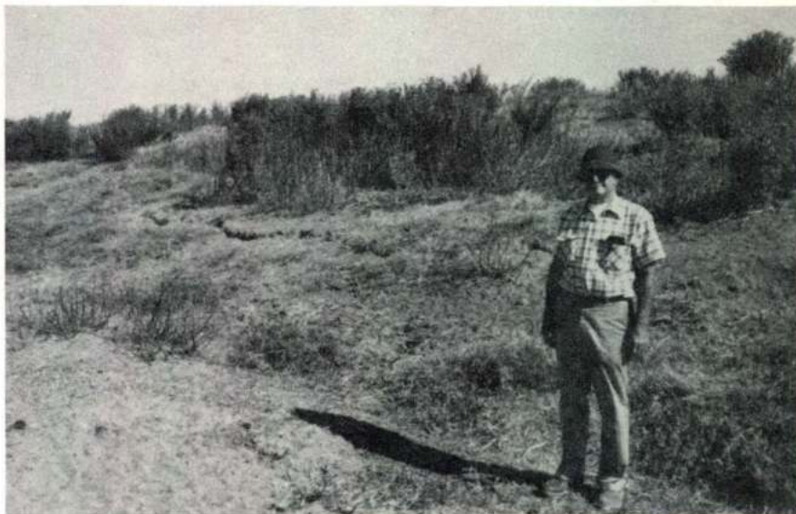
Part of the 500-foot crack that opened on the north levee of Webb Tract (Site 4) during the May 2, 1983 Coalinga earthquake. The crack was still visible two months after the earthquake when this photograph was taken.
