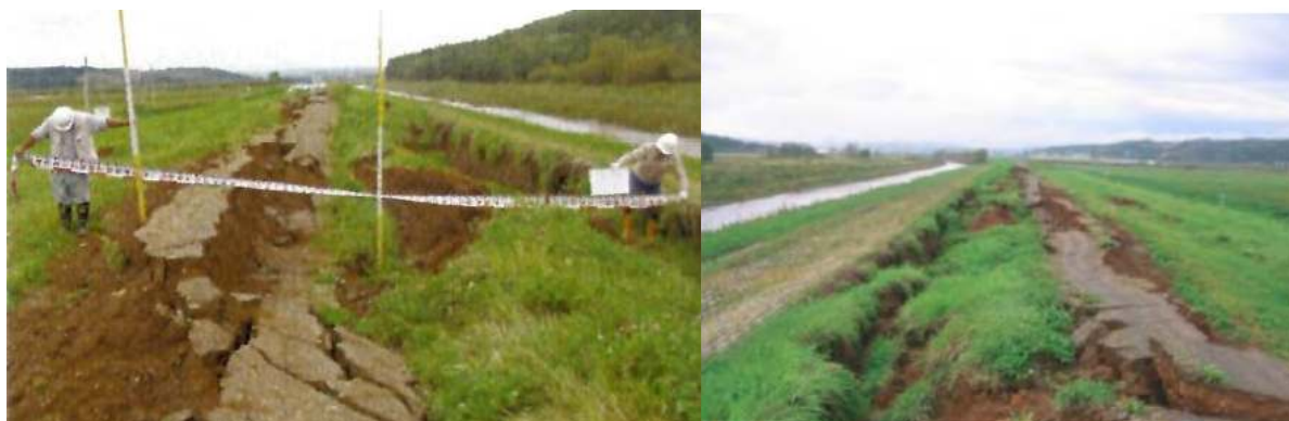
Figure 4.23 Extensive subsidence and collapse of the levee at Section 11.
