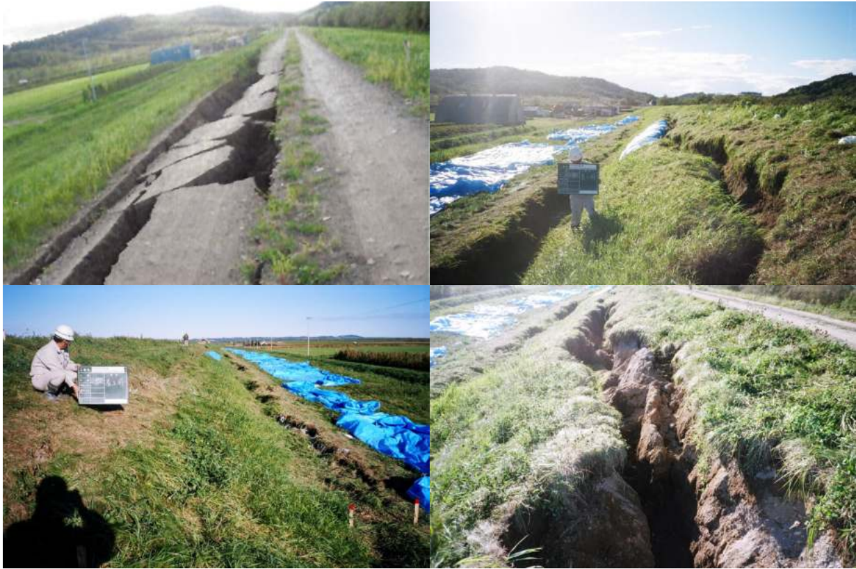
Figure 4.26 Damage at Section 12, cracks on the roadway on the levee crest (top left). Slip and displacement of the land-side slope towards the levee toe (top right, bottom).
