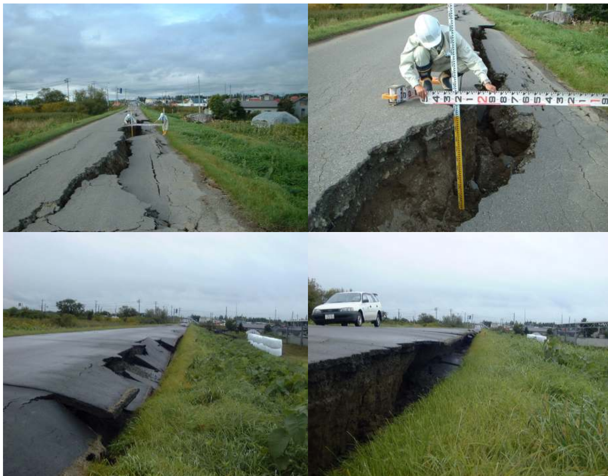
Figure 4.31 Cracks on the roadway on the levee crest at Section 14 from slip on land-side slope.
