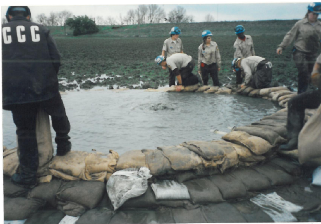
CCC crew constructing sandbag ring around boil.
