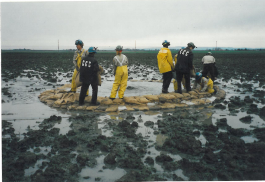
CCC crew about 1/3 of the way into boil sandbag ring.
